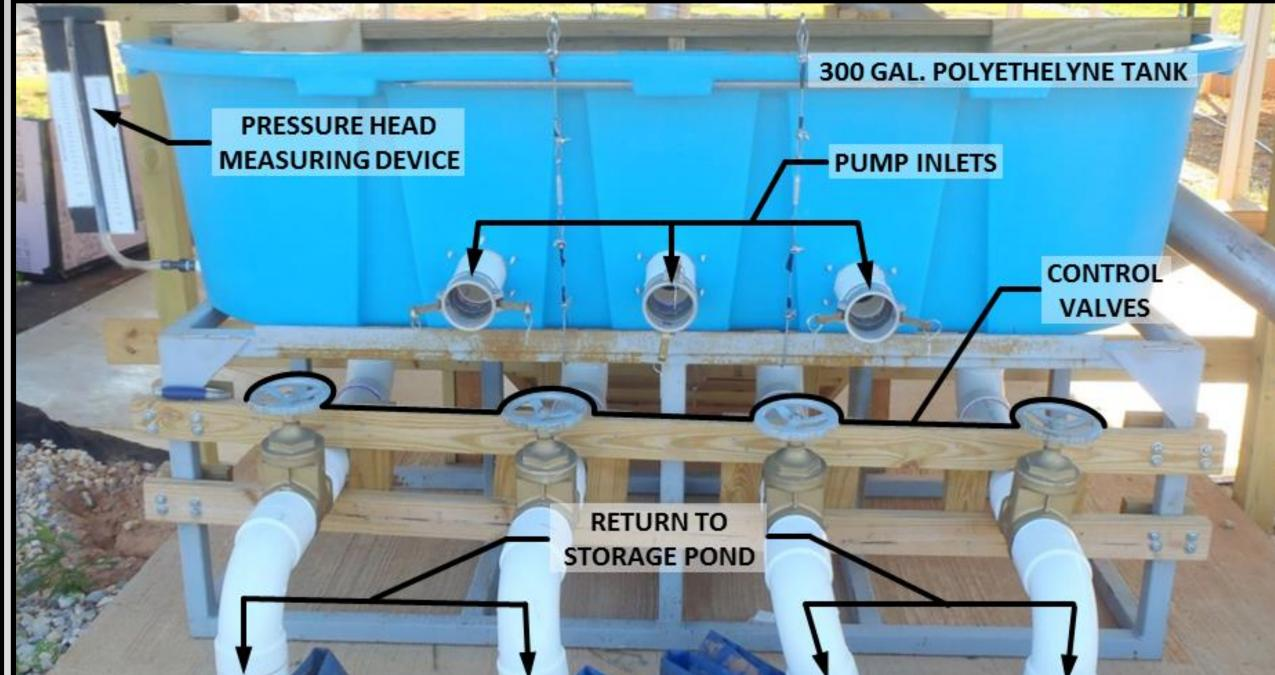
Water introduction is achieved using three semi-trash pumps. Flows are regulated using a weir plate emanating from the above tank system.
